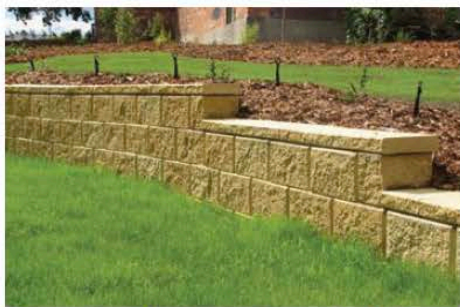
Stepping down using half corner
